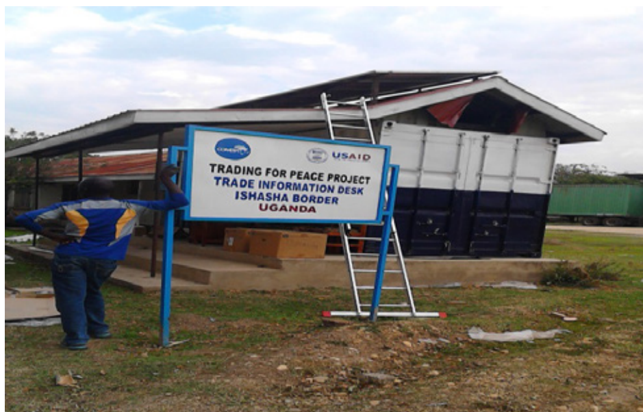
The installation of solar panels at the TID at the Ishasha border in Uganda
