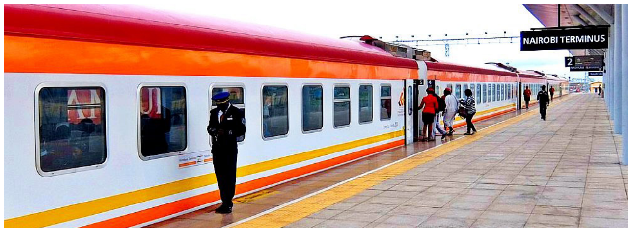
FIGURE 4: A platform at the Nairobi Terminus of the SGR
